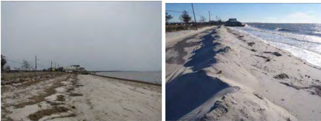
The left photograph was taken March 5, 2012 looking south. The dune was vegetated and the beach was higher in elevation compared to the post-Sandy picture on the right taken November 9, 2012. The sand in the center of the right photo has been transferred from the roadway back to the beach as a series of piles.
